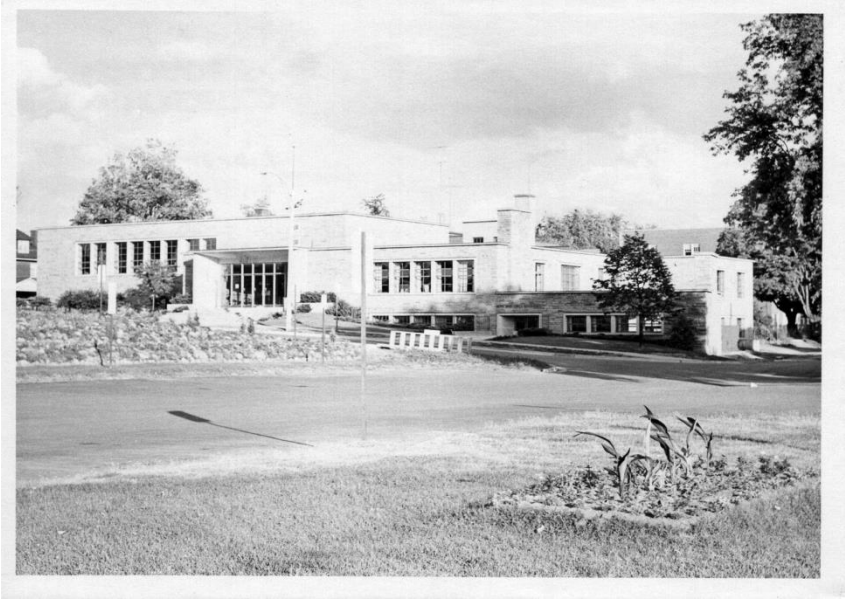
26. New Oshawa Public Library, c.1955
